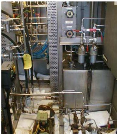
time it will become almost like resin. As the wellhead and the ESDV hydraulic systems are static (i.e. stagnant flow) contrary to ordinary hydraulic systems, which are dynamic (i.e. flow in circulation), there is a much higher risk of these resin-like sediments in components and pipes than in ordinary hydraulic systems.
