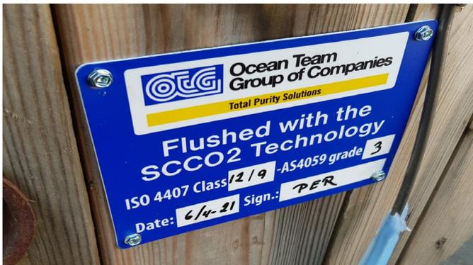
▲ Control lines flushed to a NAS class 3 before installation
