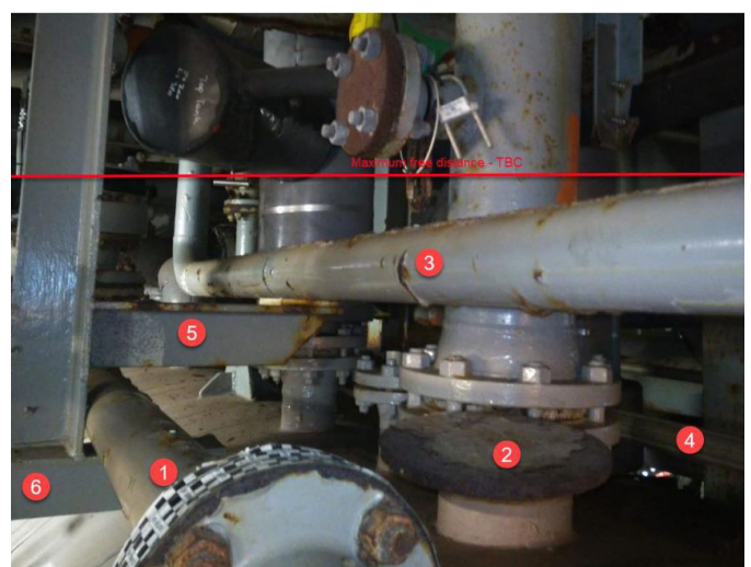
Intervention Point, Overview
